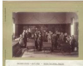
Photo of Palisade Classroom circa 1900 (1979.23.17)
