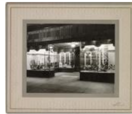
Exterior of Benge's Shoestore (2021.24.6)
