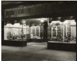
Exterior of Benge's Shoestore (2021.24.8)
