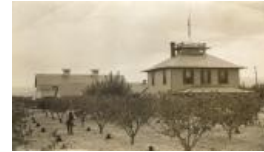
Cross Orchards House, Barn, and Orchards (1980.66.17)
