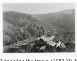
Rebuilding the tracks (1987.39.26)
