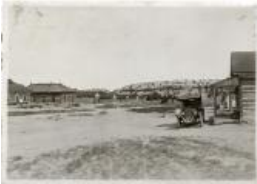
Photo of log structures with automobile (1990.8.21)
