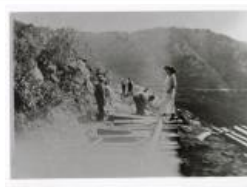
Rebuilding the Tracks (1987.39.24)
