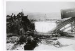
Wreck of engine #10 at bridge 2A. (1987.39.7)
