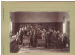
Photo of Palisade Classroom circa 1900 (1979.23.17)
