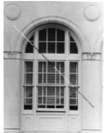
Mesa County Court House (2004.44.112)
