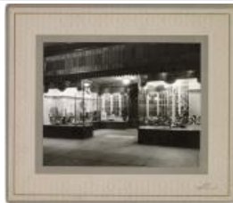
Exterior of Benge's Shoestore (2021.24.6)
