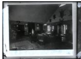
Interior of the Uintah Hotel (2023.40.47)
