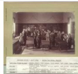
Photo of Palisade Classroom circa 1900 (1979.23.17)
