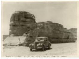
Highway built by CCC (1982.135.5)
