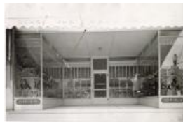
Exterior of the Benge's Shoe store (2021.24.11)
