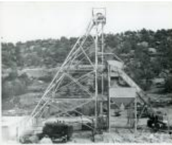
Steel headframe and ore bins at Colorado Plateau. Vertical Shaft operations. (1983.63.176)
