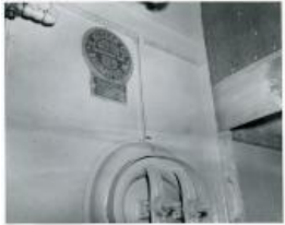
Grand Junction boiler House AEC Compound (1983.63.112)
