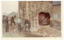
Base of stack (1983.63.50)
