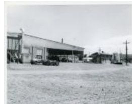
AEC Sampling Plant Expansion site (23 Jul 1956) (1983.63.139)
