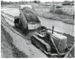
Dump truck unloading fill on dike (1983.63.4)
