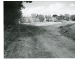
Gunnison River Bridge and dike (Black Bridge) (1983.63.17)
