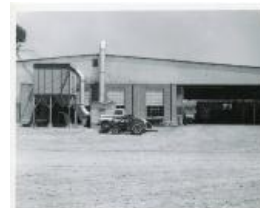
AEC Sampling Plant Expansion site (23 Jul 1956) (1983.63.140)
