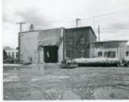
AEC Heating Plant (May 1957) (1983.63.125)
