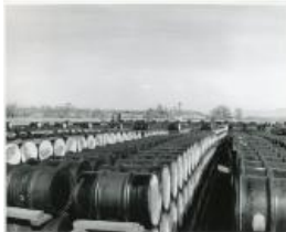
Vanadium storage closeup view looking Northwest (1983.63.158)
