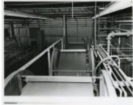
Pilot Plant - Grand Junction (1983.63.132)
