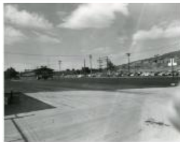
Grand Junction Compound paving parking lot (9 July 1957) [Duplicate] (1983.63.108)
