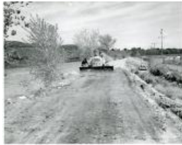
Two CAT bulldozers working on dike (1983.63.10)
