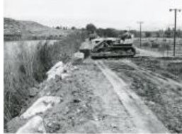
CAT bulldozer pushing riprap into river bank (1983.63.7)
