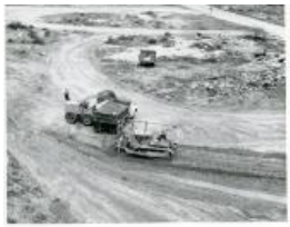
Loading fill for dike across road from AEC compound (1983.63.11)
