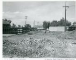
Getting sampling plant expansion slab area ready for pour (1983.63.146)
