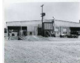
AEC Sampling Plant Expansion site (23 Jul 1956) (1983.63.142)
