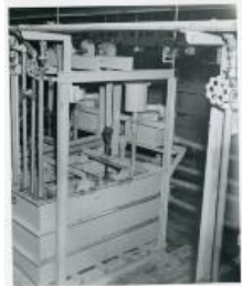
Pilot Plant - Grand Junction (1983.63.135)
