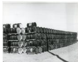
Vanadium storage looking Northwest - 55 drums comparatively new (note rust on bottom and stacking arrangement) (18 Feb 1958) (1983.63.160)
