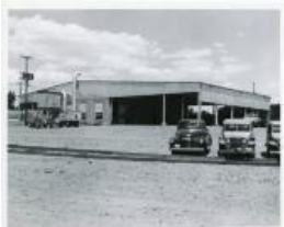
AEC Sampling Plant Expansion site (23 Jul 1956) (1983.63.141)
