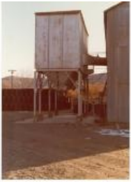
Silo with drums in background (1983.63.231)
