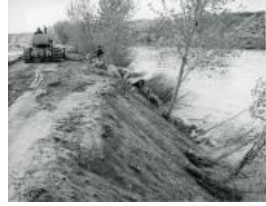
Photo of CAT Bulldozer working on dike along Gunnison River (1983.63.3)
