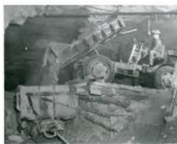
Underground dumping ore from diesel dump truck into Granby type car (1983.63.183)
