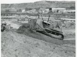
CAT Bulldozer pushing up fill across road (1983.63.12)
