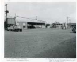
AEC Sampling Plant Expansion site (23 Jul 1956) (1983.63.143)
