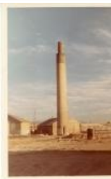
Stack standing with buildings (1983.63.51)
