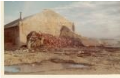
Large pile of rubble (Photo) (1983.63.59)
