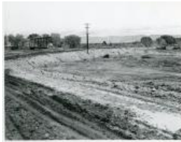
Gunnison Bridge and dike (1983.63.9)
