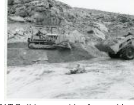
CAT Bulldozer and loader working on fill (1983.63.13)
