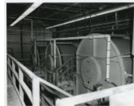
Pilot Plant - Grand Junction (1983.63.133)
