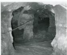
Pillar supported stopes in an underground Uranium mine. Pillars and ore will be extracted in retreat mining. (1983.63.181)
