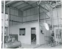
New boiler house building (1956) (1983.63.113)
