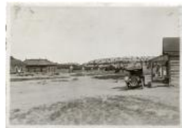
Photo of log structures with automobile (1990.8.21)
