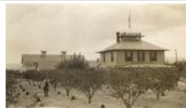
Cross Orchards House, Barn, and Orchards (1980.66.17)
