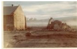
Stack base in pile, building (Photo) (1983.63.58)
