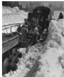
Rerailment, Cumbres Pass (1997.8.2)
