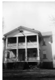
House in Pine Creek Township (1983.55.5)
