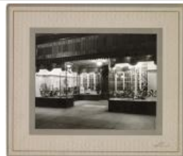
Exterior of Benge's Shoestore (2021.24.6)
