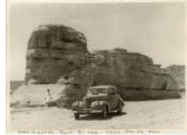
Highway built by CCC (1982.135.5)
