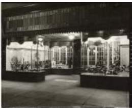
Exterior of Benge's Shoestore (2021.24.8)
