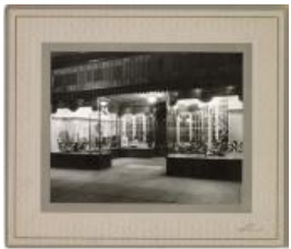
Exterior of Benge's Shoestore (2021.24.6)
