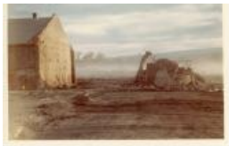
Stack base in pile, building (Photo) (1983.63.58)
