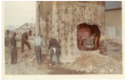
Base of stack (1983.63.50)
