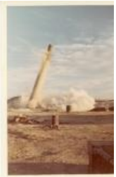
Stack starting to fall (Photo) (1983.63.54)
