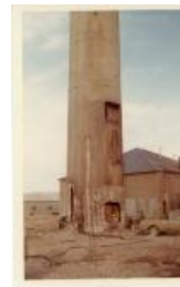
Climax uranium stack demolition 24 Nov 1970 (old sugar factory area) (1983.63.49)
