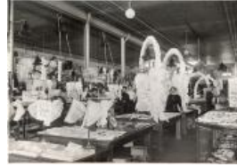
Photo and negative, Interior of the Fair Store (1999.8.34)
