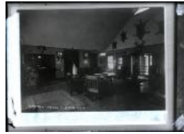
Interior of the Uintah Hotel (2023.40.47)
