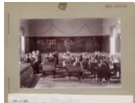
Photo of Palisade Classroom circa 1900 (1979.23.8)
