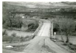
Photo of The State Bridge crossing a river (1987.26.55)
