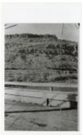
Photo of bridge by Rapid Creek (2019.2.61)
