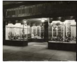
Exterior of Benge's Shoestore (2021.24.8)
