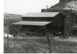
Photo of the Pyeatt barn (1987.26.39)
