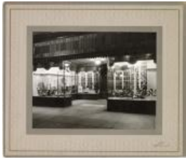
Exterior of Benge's Shoestore (2021.24.6)
