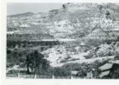
Photo of Ute Water Plant with surrounding landscape (1987.26.15)
