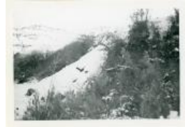
Photo of Blue Flame Mine remnants (1987.26.46)
