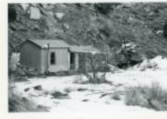
Photo of Winger Mine and structure (1987.26.48)
