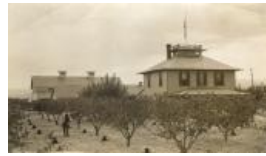
Cross Orchards House, Barn, and Orchards (1980.66.17)
