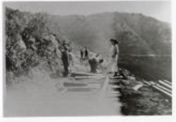
Rebuilding the Tracks (1987.39.24)
