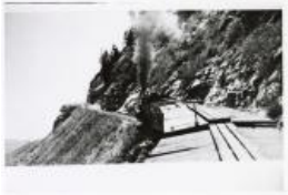
Uintah locomotive climbing 7.5% grade on Baxter Pass. (1987.39.5)
