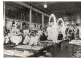
Photo and negative, Interior of the Fair Store (1999.8.34)
