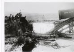
Wreck of engine #10 at bridge 2A. (1987.39.7)
