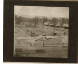
Fair Store Construction (1999.8.37)
