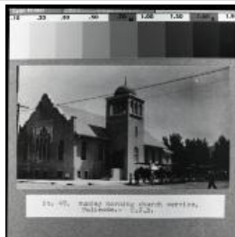
Methodist Church in Palisade (1980.115.47)
