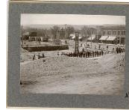
Fair Store Construction (1999.8.38)
