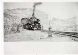
Mallet #51 crossing bridge into Atchee. (1987.39.15)
