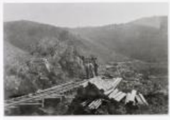
Rebuilding the tracks (1987.39.26)
