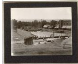
Fair Store Construction (1999.8.36)
