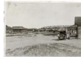
Photo of log structures with automobile (1990.8.21)
