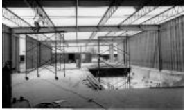
The Daily Sentinel Press Plant (2004.44.668)
