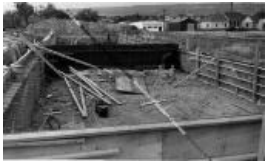
The Daily Sentinel Press Plant (2004.44.660)
