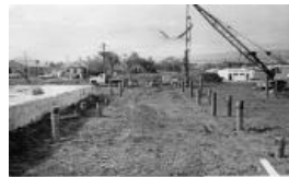
The Daily Sentinel Press Plant (2004.44.654)
