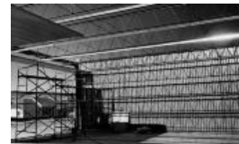
The Daily Sentinel Press Plant (2004.44.667)
