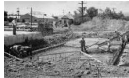
The Daily Sentinel Press Plant (2004.44.662)
