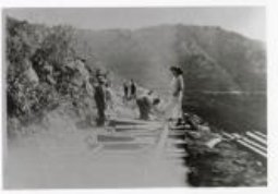
Rebuilding the Tracks (1987.39.24)
