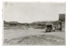
Photo of log structures with automobile (1990.8.21)
