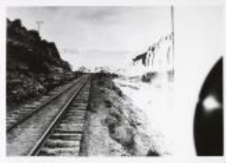
Uintah crossing bridge into Watson, Utah (1987.39.3)
