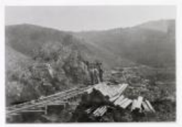
Rebuilding the tracks (1987.39.26)
