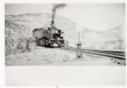
Mallet #51 crossing bridge into Atchee. (1987.39.15)
