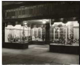
Exterior of Benge's Shoestore (2021.24.8)
