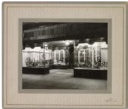
Exterior of Benge's Shoestore (2021.24.6)
