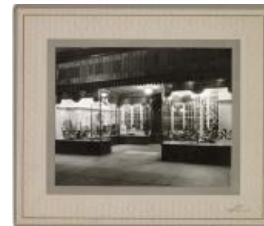
Exterior of Benge's Shoestore (2021.24.6)
