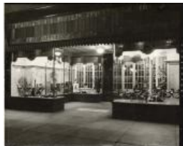
Exterior of Benge's Shoestore (2021.24.8)
