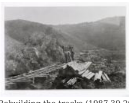
Rebuilding the tracks (1987.39.26)
