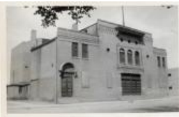
Photo of Park Opera House (2022.0.3)
