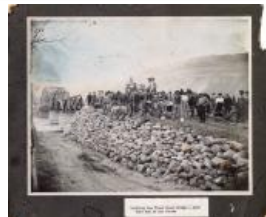
Photo of the Construction of Palisade's First Steel Bridge (1979.23.123)
