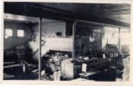
Photo and negative of Fair building, cashier's gallery (1999.8.9)
