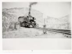
Mallet #51 crossing bridge into Atchee. (1987.39.15)
