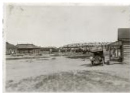
Photo of log structures with automobile (1990.8.21)
