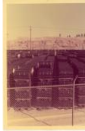
Rows of drums looking East (1983.63.38)
