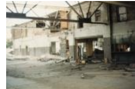
Color Photo of the demolition of Western Slope Auto (1987.89.11)
