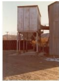
Silo with drums in background (1983.63.231)
