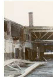
Color Photo of the demolition of Western Slope Auto (1987.89.22)
