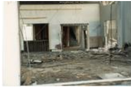
Color Photo of the demolition of Western Slope Auto (1987.89.7)
