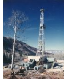
Astral Oil Co.'s Drilling Rig at Rulison (2HA161.10)
