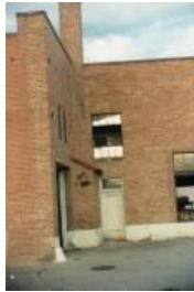
Photo of the demolition of Western Slope Auto (1987.89.1)
