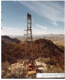
Core Drilling Photograph (1983.78.3)
