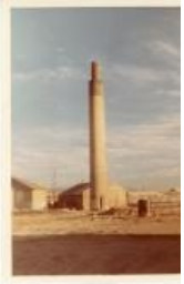
Stack standing with buildings (1983.63.51)
