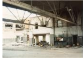
Color Photo of the demolition of Western Slope Auto (1987.89.24)
