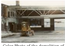
Color Photo of the demolition of Western Slope Auto (1987.89.20)
