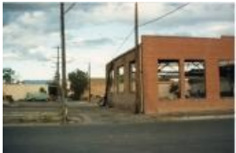
Color Photo of the demolition of Western Slope Auto (1987.89.5)
