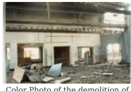
Color Photo of the demolition of Western Slope Auto (1987.89.17)
