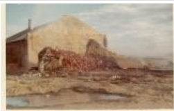
Large pile of rubble (Photo) (1983.63.59)
