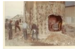
Base of stack (1983.63.50)
