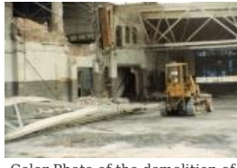
Color Photo of the demolition of Western Slope Auto (1987.89.21)
