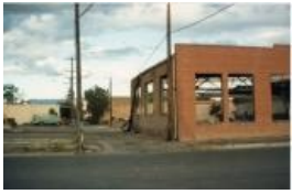
Color Photo of the demolition of Western Slope Auto (1987.89.5)
