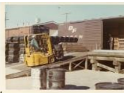
Hyster operator carrying two drums up ramp for loading in freight car (1983.63.34)
