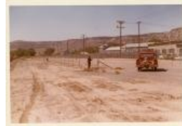
Barbwire East side of AEC Compound + negative (1983.63.204)
