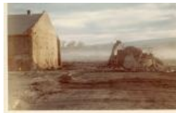
Stack base in pile, building (Photo) (1983.63.58)
