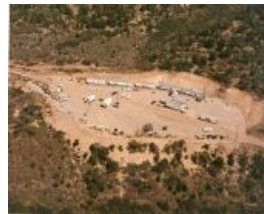
Project Rulison Parking Area (2HA161.6)
