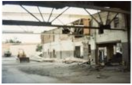
Color Photo of the demolition of Western Slope Auto (1987.89.12)
