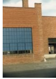
Color Photo of the demolition of Western Slope Auto (1987.89.3)
