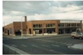
Color Photo of the demolition of Western Slope Auto (1987.89.6)
