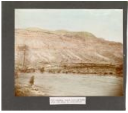
Photo of Palisade's Old Pumping Plant (1979.23.115)
