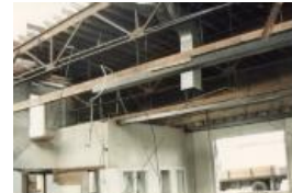
Color Photo of the demolition of Western Slope Auto (1987.89.8)
