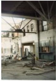
Color Photo of the demolition of Western Slope Auto (1987.89.13)
