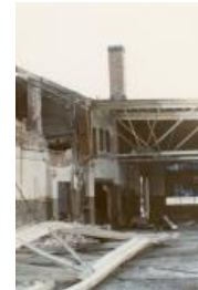
Color Photo of the demolition of Western Slope Auto (1987.89.22)
