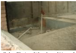
Color Photo of the demolition of Western Slope Auto (1987.89.16)
