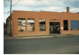
Color Photo of the demolition of Western Slope Auto (1987.89.4)
