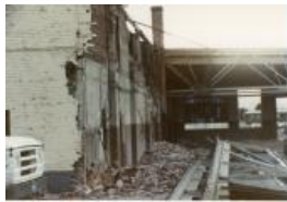
Color Photo of the demolition of Western Slope Auto (1987.89.18)
