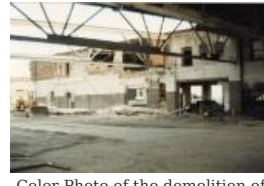
Color Photo of the demolition of Western Slope Auto (1987.89.15)
