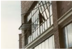
Color Photo of the demolition of Western Slope Auto (1987.89.10)
