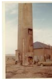
Climax uranium stack demolition 24 Nov 1970 (old sugar factory area) (1983.63.49)
