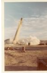
Stack starting to fall (Photo) (1983.63.54)
