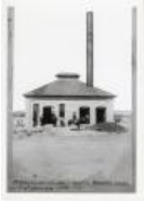
Powerhouse of First Water Works (F224.3)
