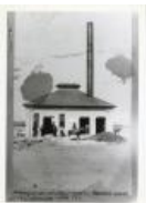
Powerhouse of First Water Works [Duplicate] (F224.2)
