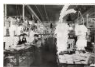
Photo and negative, Interior of the Fair Store (1999.8.35)
