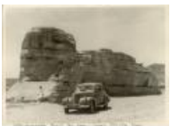
Highway built by CCC (1982.135.5)
