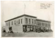
Photo of the Corner of Main and Third St., Palisade (1979.23.100)
