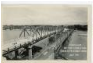
5th Street Bridge (2004.44.156)
