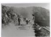
Rebuilding the Tracks (1987.39.24)
