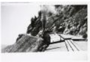
Uintah locomotive climbing 7.5% grade on Baxter Pass. (1987.39.5)
