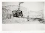
Mallet #51 crossing bridge into Atchee. (1987.39.15)
