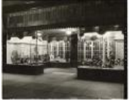
Exterior of Benge's Shoestore (2021.24.8)
