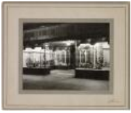
Exterior of Benge's Shoestore (2021.24.6)
