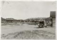
Photo of log structures with automobile (1990.8.21)
