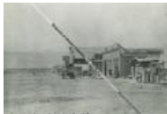
Main Street, Looking West (2004.44.790)
