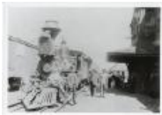
Photo of narrow gauge locomotive No. 164 at depot (1990.10.39)
