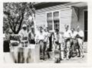
Jaycee Nursery Being Built (1979.45.2)
