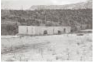
B&W photo of J.P. Hawlow's stone house on a hillside (1987.38.20)
