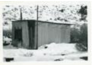
Photo of structure at Winger Mine (1987.26.47)
