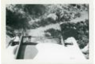
Photo of snow covered equipment above road (1987.26.13)
