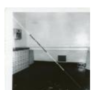
Interior of building #20 AEC Compound AS & R C. Laboratory 19 Dec 1952 (Photo) (1983.63.62)
