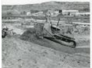
CAT Bulldozer pushing up fill across road (1983.63.12)
