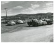
Grand Junction Compound paving parking lot (9 July 1957) (1983.63.107)
