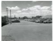
Grand Junction Compound parking lot prior to black topping (18 June 1957) (1983.63.100)
