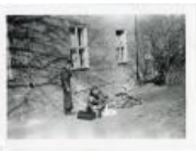
Two Soldiers in Front of Building (2023.30.8)
