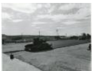
Grand Junction Compound paving parking lot (9 July 1957) (1983.63.106)
