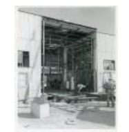
New boiler house outside looking in (1956) (1983.63.114)
