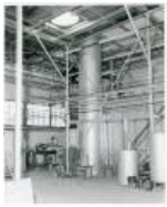
Grand Junction AEC Compound Boiler house inside (26 Sep 1956) (1983.63.116)
