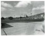
Grand Junction Compound paving parking lot (9 July 1957) [Duplicate] [Duplicate] (1983.63.109)
