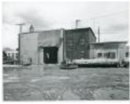
AEC Heating Plant (May 1957) (1983.63.125)
