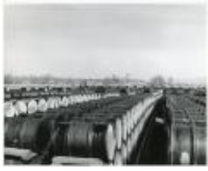
Vanadium storage closeup view looking Northwest (1983.63.158)
