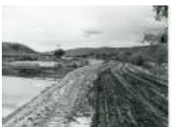
Dike between compound and Gunnison River (1983.63.5)
