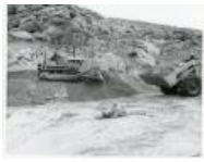
CAT Bulldozer and loader working on fill (1983.63.13)
