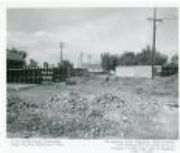
Getting sampling plant expansion slab area ready for pour (1983.63.146)
