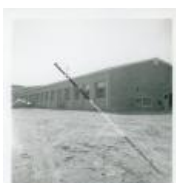
Outside of building AEC (Photo) (1983.63.68)
