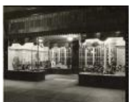
Exterior of Benge's Shoestore (2021.24.8)
