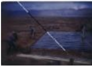
Slide: Anomaly at Walker Field Airport (1983.63.22)
