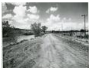
Dike along Gunnison River (1983.63.14)
