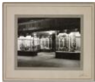
Exterior of Benge's Shoestore (2021.24.6)
