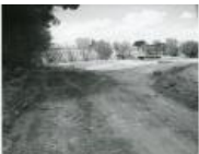
Gunnison River Bridge and dike (Black Bridge) (1983.63.17)
