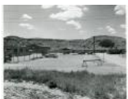
Grand Junction Compound parking lot prior to black topping (18 June 1957) [Duplicate] [Duplicate] [Duplicate] (1983.63.105)
