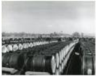
Vanadium storage closeup view looking Northwest (Copy of 158) (1983.63.159)
