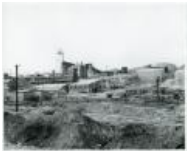
Uranium processing mill at Monticello, Utah. This is the only government owned uranium mill. (1983.63.188)
