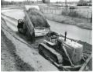
Dump truck unloading fill on dike (1983.63.4)
