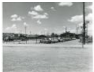
Grand Junction Compound parking lot prior to black topping (18 June 1957) (1983.63.102)
