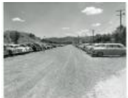
Grand Junction Compound parking lot prior to black topping (18 June 1957) (1983.63.101)
