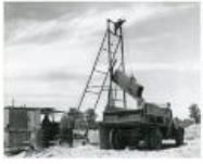
Headframe and skip hoist at small uranium mine. This is an inclined shaft mine. (1983.63.187)
