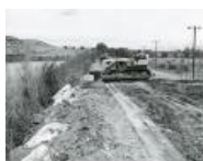
CAT bulldozer pushing riprap into river bank (1983.63.7)
