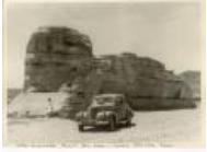
Highway built by CCC (1982.135.5)
