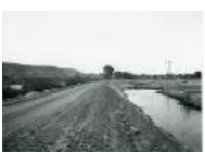
Dike along Gunnison River (1983.63.6)
