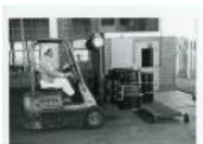
Last load forklift moving drums - Daily Sentinel Photo + 1 (1983.63.166)
