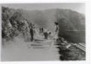
Rebuilding the Tracks (1987.39.24)
