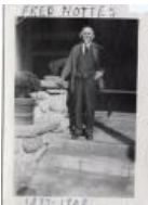
Photograph of Fred Hottes (1979.23.16)
