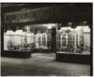
Exterior of Benge's Shoestore (2021.24.8)
