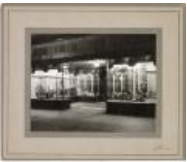
Exterior of Benge's Shoestore (2021.24.6)
