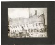
Black and white photo of building construction (1987.75.5)
