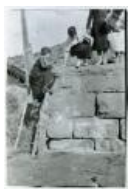
Photograph of Ann Stokes on Rapid Creek Bridge (1986.25.5)
