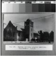
Methodist Church in Palisade (1980.115.47)
