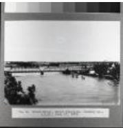
Grand River channel (Colorado River) and 5th Street Bridge (1980.115.2)
