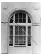
Mesa County Court House (2004.44.112)
