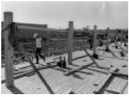
Building the new Sentinel (2004.44.704)
