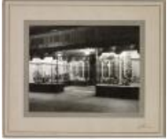
Exterior of Benge's Shoestore (2021.24.6)
