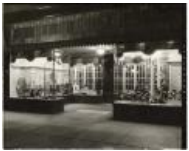
Exterior of Benge's Shoestore (2021.24.8)
