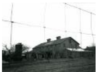
Photo of the Cross Orchards Barn (2008.67.7)
