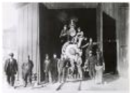
Employees of the Uintah Railway at Atchee (1986.0.3.40)
