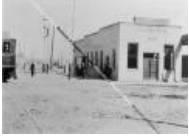
GJ & GRV substation (1995.82.10)
