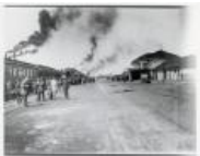
Grand Junction Railroad Station & Yards, 1900-1920 (F720.57)
