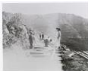
Bridge and building crew. (1987.39.25)
