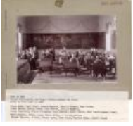
Photo of Palisade Classroom circa 1900 (1979.23.8)
