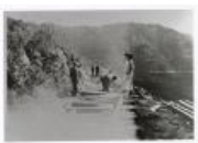
Rebuilding the Tracks (1987.39.24)
