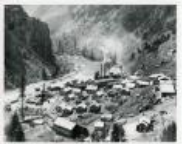
Construction Camp in Black Canyon (2004.44.76)
