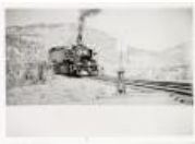
Mallet #51 crossing bridge into Atchee. (1987.39.15)
