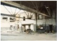
Color Photo of the demolition of Western Slope Auto (1987.89.24)
