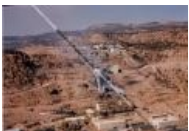
Uranium Vanadium Mine at Uravan (2006.141.3)
