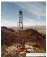
Core Drilling Photograph (1983.78.3)
