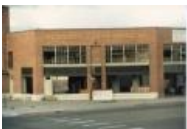
Color Photo of the demolition of Western Slope Auto (1987.89.23)
