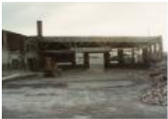
Color Photo of the demolition of Western Slope Auto (1987.89.19)
