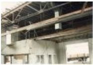
Color Photo of the demolition of Western Slope Auto (1987.89.8)
