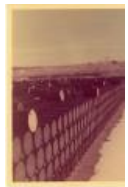
AEC Compound uranium concentrate drum storage (1983.63.35)
