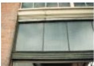
Color Photo of the demolition of Western Slope Auto (1987.89.9)
