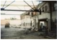
Color Photo of the demolition of Western Slope Auto (1987.89.14)
