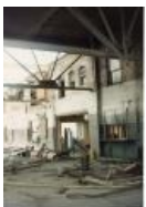
Color Photo of the demolition of Western Slope Auto (1987.89.13)
