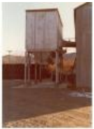
Silo with drums in background (1983.63.231)
