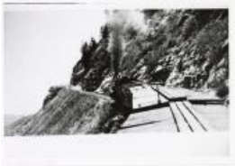
Uintah locomotive climbing 7.5% grade on Baxter Pass. (1987.39.5)
