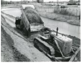
Dump truck unloading fill on dike (1983.63.4)
