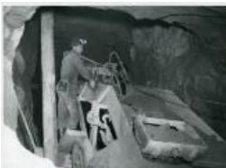
In Colorado Plateau Uranium Mine, scrapping up ore on moveable scraper loading slide into mine car (1983.63.175)
