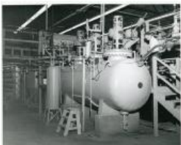
Alkaline Leach Autoclave - Pilot Plant, Grand Junction (1983.63.136)
