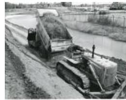
Dump truck unloading fill on dike (1983.63.4)
