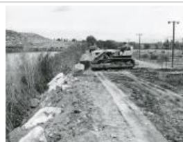
CAT bulldozer pushing riprap into river bank (1983.63.7)
