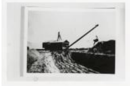
Highline Canal Steam Powered Dragline (F462.1)
