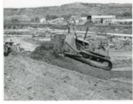
CAT Bulldozer pushing up fill across road (1983.63.12)
