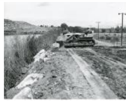
CAT bulldozer pushing riprap into river bank (1983.63.7)
