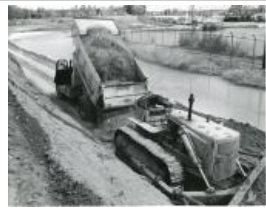
Dump truck unloading fill on dike (1983.63.4)
