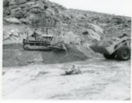
CAT Bulldozer and loader working on fill (1983.63.13)
