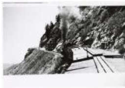
Uintah locomotive climbing 7.5% grade on Baxter Pass. (1987.39.5)
