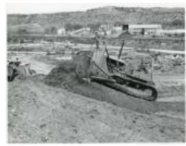
CAT Bulldozer pushing up fill across road (1983.63.12)
