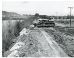
CAT bulldozer pushing riprap into river bank (1983.63.7)
