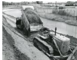
Dump truck unloading fill on dike (1983.63.4)
