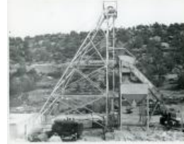
Steel headframe and ore bins at Colorado Plateau. Vertical Shaft operations. (1983.63.176)
