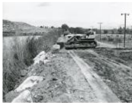
CAT bulldozer pushing riprap into river bank (1983.63.7)
