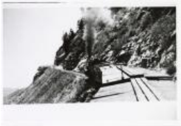
Uintah locomotive climbing 7.5% grade on Baxter Pass. (1987.39.5)
