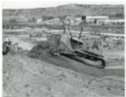
CAT Bulldozer pushing up fill across road (1983.63.12)
