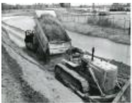
Dump truck unloading fill on dike (1983.63.4)
