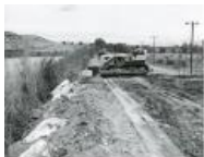
CAT bulldozer pushing riprap into river bank (1983.63.7)
