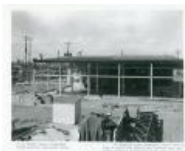
Starting construction SS Sampling plant expansion south dock showing new concrete slab (4 Sep 1956) (1983.63.145)
